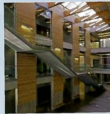
Atrium & inter-connecting staircase, Kwantlen University College Library.
